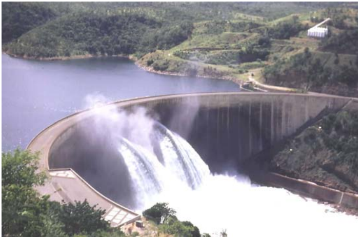
Kariba Dam, on the Zambezi
