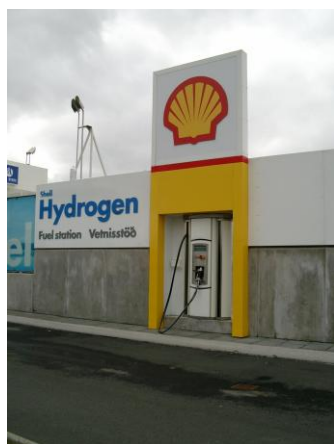
Hydrogen filling station, Reykjavik
