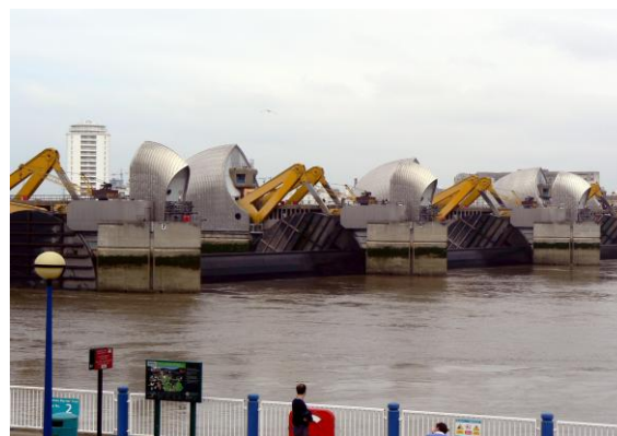
Thames Barrier, gates being raised during monthly tests
