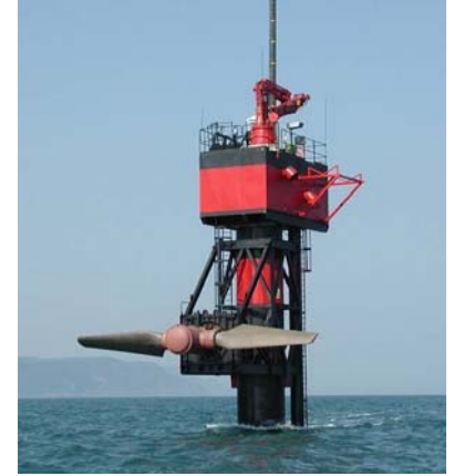
Fig 2 The Seaflow turbine raised for maintenance
