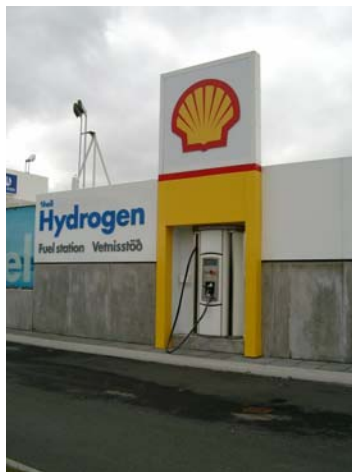
Hydrogen filling station, Reykjavik
